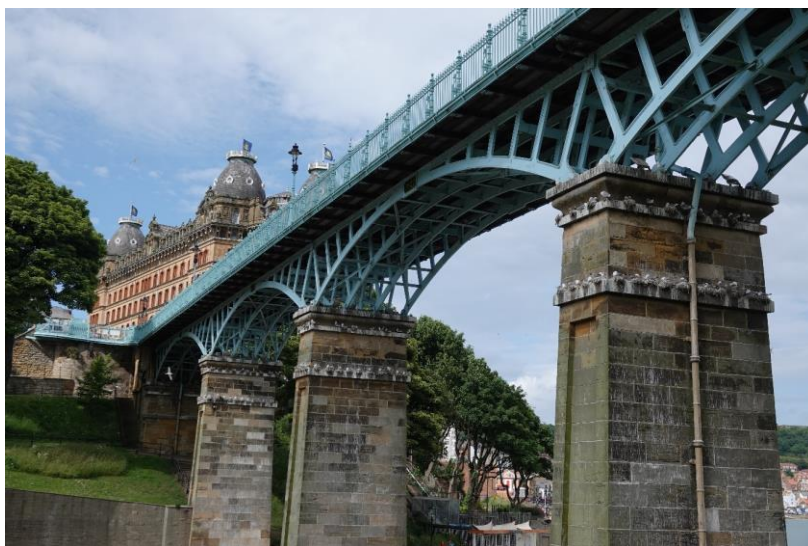
Spa Bridge Scarborough. Photo: Nick Addey.
