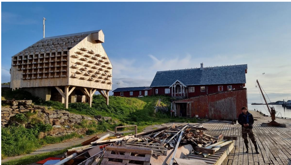
Figure 3. The Kittiwake hotel at Kårøya on 10 June 2025, when nest platforms had also been mounted on the seafront wall. The building in the background is Nilssenhuset, featuring its new roof. © Tycho Anker-Nilssen.
